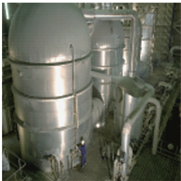
Fig.6 Multi-effect evaporators
